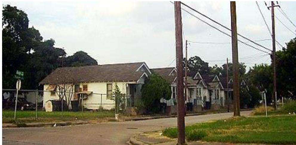
Fig 17. No paints on the road and roads need repair works
