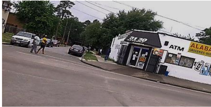
Fig 14. Some of the roads do not have paints or traffic signs
