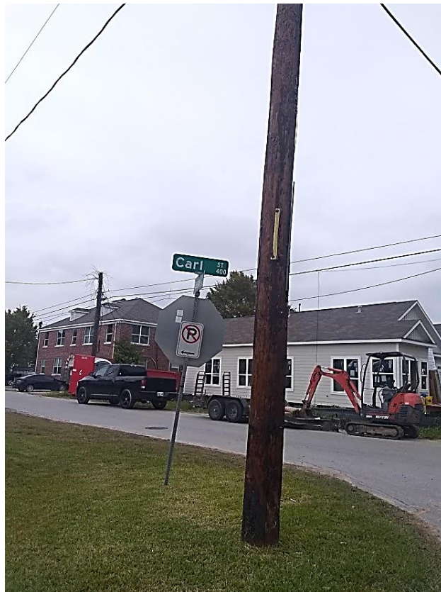
Fig 8. Clearing ground to install new sidewalks.
