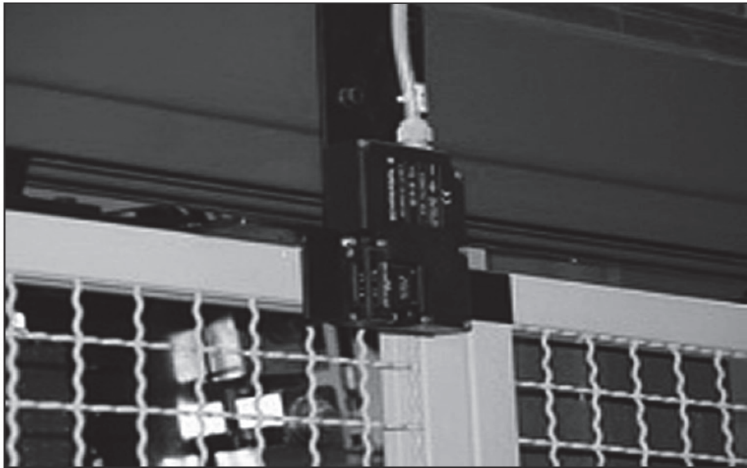
Fig 5. Interlock switch on sliding gate [7]
